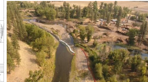
Bird Track Springs Construction September 2018
